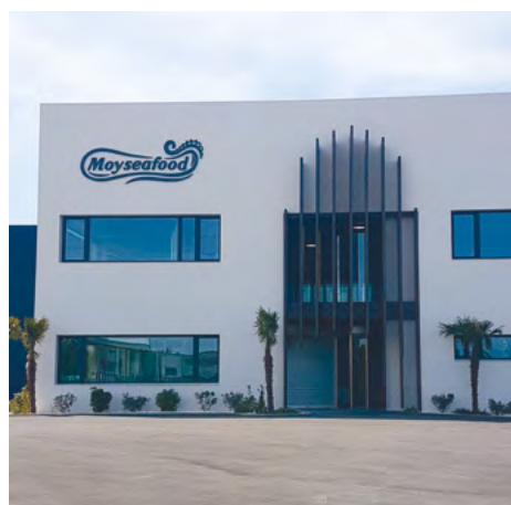
Industrial building enclosing, Cádiz, Spain
