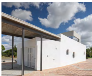
Comercial building, Cádiz
